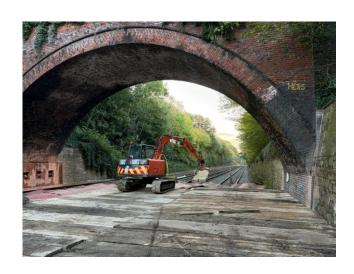
The photos show a similar methodology, where Flying Arch bridge was demolished on 4-5 October 2025 using excavators during a 54hr period. The demolition of Kirk Hill bridge will be done in the same timeframe.
